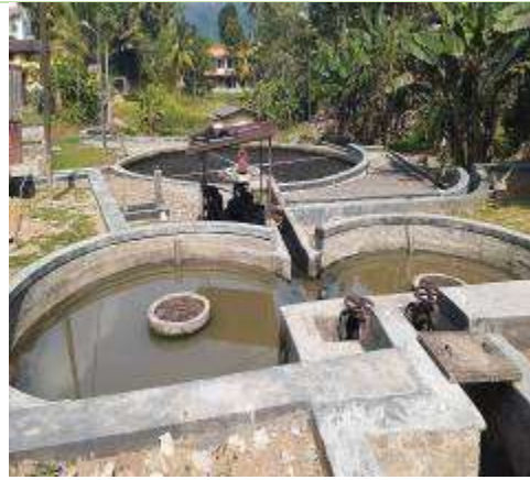
Site visit to the waste water treatment plant
