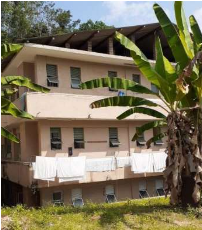
Existing building allocated for the proposed construction
